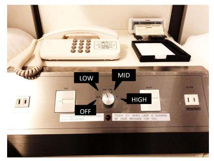
①Turn on the switch and adjust the air flow. OFF:OFF L:LOW M:MID H:HIGH
